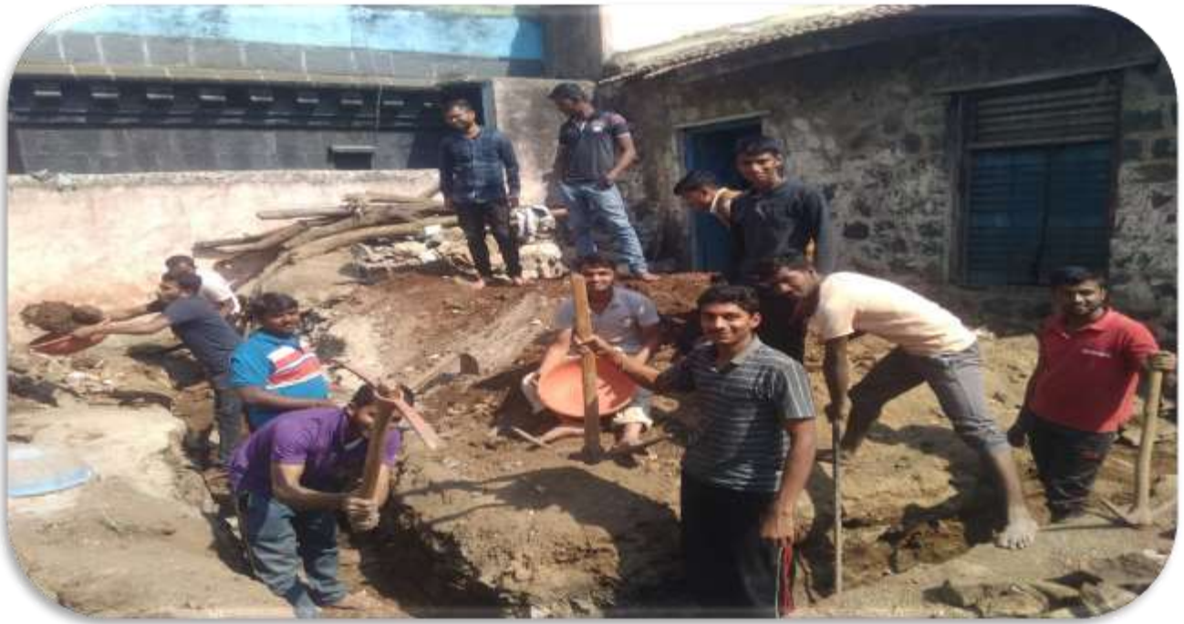
Foundation of primary school
